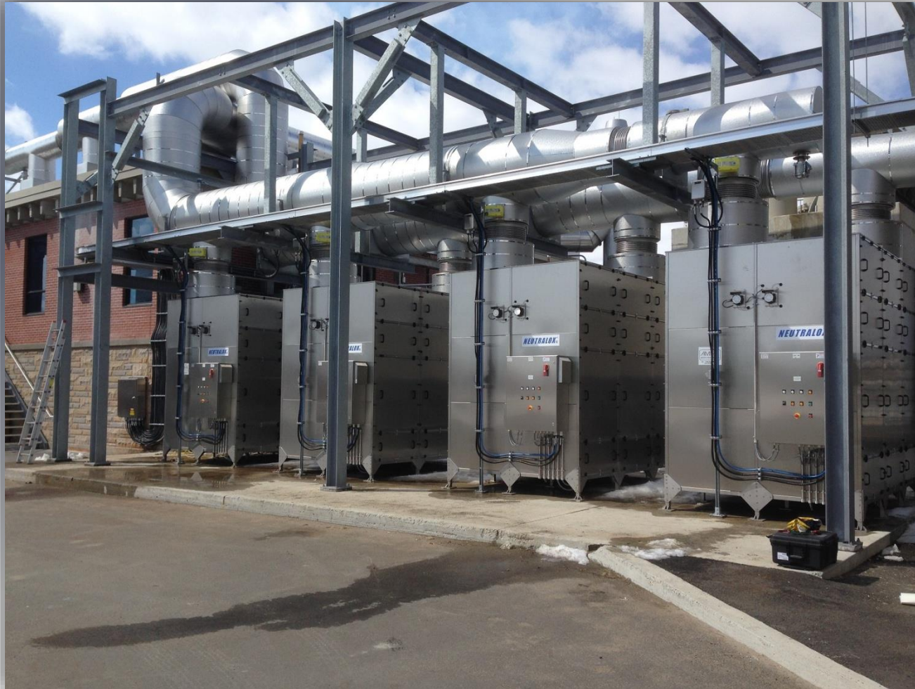
Sudbury headworks and pumping station, H 2 S
