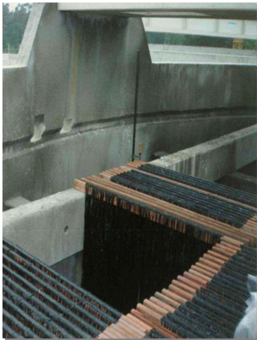
Concrete support structure
