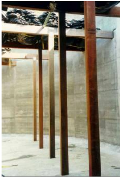
Wood support structure
