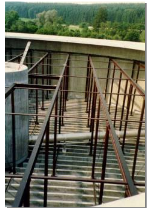
Steel support structure
